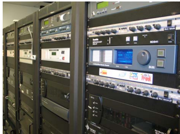
Fig. 5: Backwards Compatibility. Two generations of broadcast facility remote control equipment at a central studio facility in Hooksett, NH. Photo courtesy of Dirk Nadon, Director of Engineering NH, Nassau Broadcasting.
